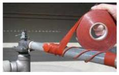
Various heat-resistant material tapes are available for fixing the heater.
